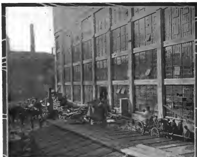
At the Dayton Electric Laboratory Co., Dayton, O., after the flood. Donkey engine and fire engine pumping
